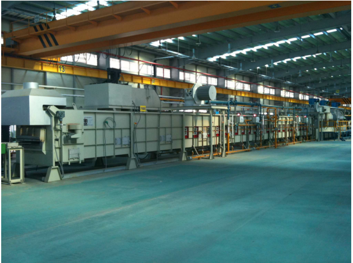
FIB Belgium: le four avant...
